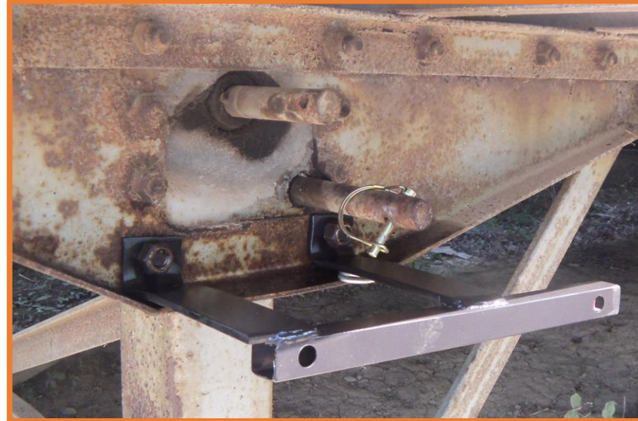
Trailer Bar Installed
